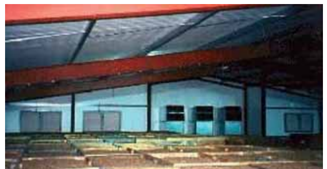
Internal view of loaded potato box store with large roof space important for crop inspection and even air distribution
