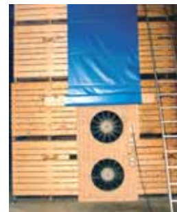
A Dutch curing system. Air is forced through the bins by fans, similar to forced air cooling.
