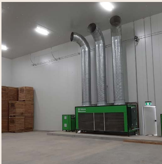
Figure 20. The Tolsma drying wall for curing freshly harvested/cut seed potatoes (left) and the Tolsma open space ventilation and cooling system (right). Images supplied by Tolsma.
