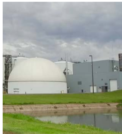
At Cavendish Farms on Prince Edward Island, digesters break down potato waste, producing biogas that fuels the boilers in the company's nearby French fry processing facility. (Image: Pat Martel/CBC)
