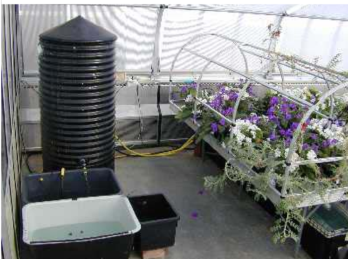
Figure 34 Sand filtration system – Plant Research Centre
